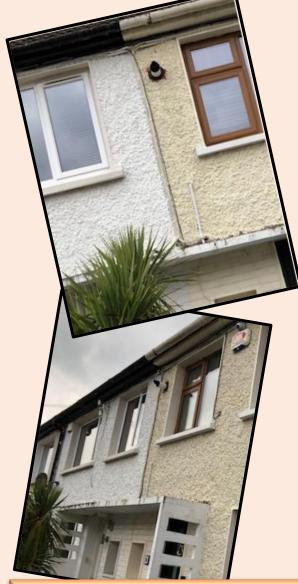
An RGI when carrying out an Annual Service found that the Condense Pipe from the High Efficiency Boiler was terminating directly onto the roof of a porch.
