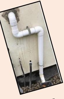
Here is an example of where an RGI had taken the necessary steps to increase the size of the condense pipework to 32mm. However, he utilised three 90° bends externally where one 90° bend with an offset or a 45° bend would have sufficed on the downpipe section would have sufficed.
