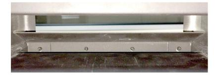
Missing or worn rivets – the appliance can be affected by rivets where the head has been broken off or the rivet is missing completely.
